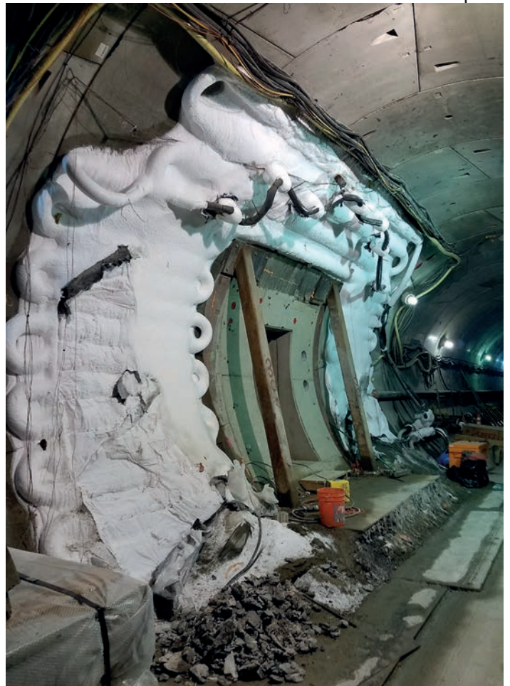
Above: Figure 3, Artificial ground freezing used in cross passage construction PHOTO COURTESY OF SOILFREEZE INC
